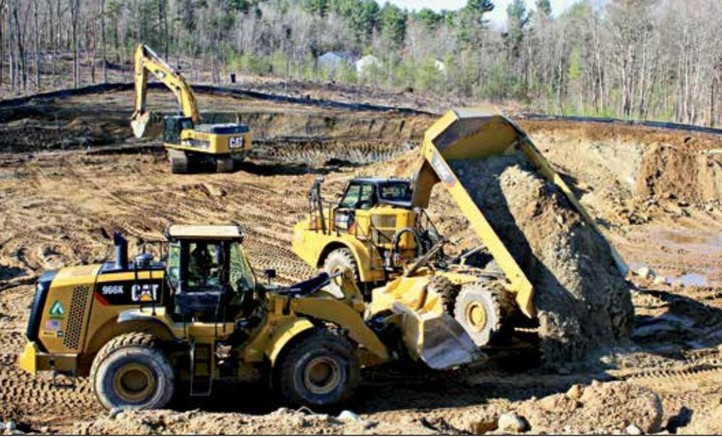
A CAT 966 Loader waits to spread excavated material deposited by a CAT 735C Off-Highway Truck as a CAT excavator works in background.
