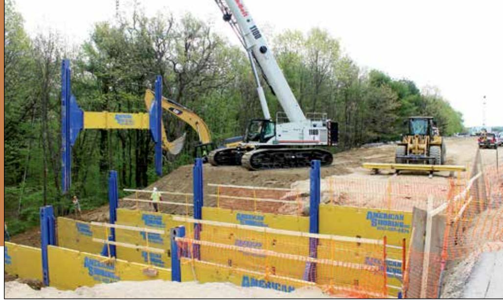
A Link-Belt TCC1100 Crane helps assemble components for American Shoring's double wall slide-rail system being used to support trench for 12-foot by 12-foot box culvert pedestrian underpass.
