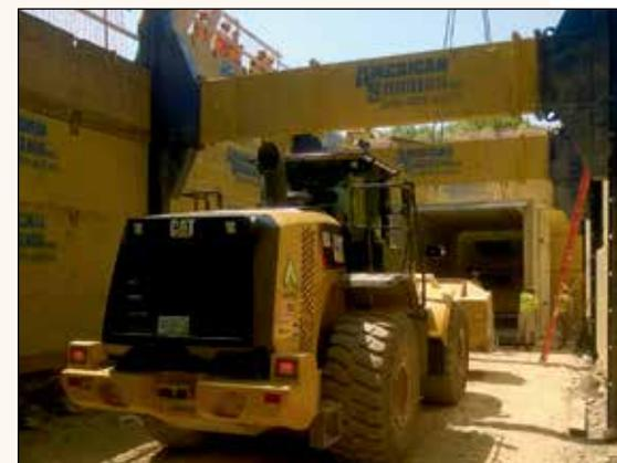
Inside shoring, a CAT 966 Loader passes beneath rolling strut to push culvert sections together.
